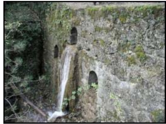
Figure 2.6. Check dam in 2005
