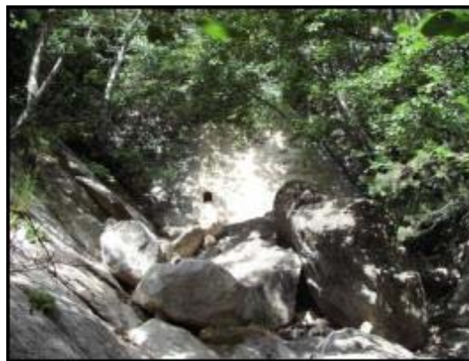
Figure 2.2. Check dam base to correction of left branch (November 2004).
