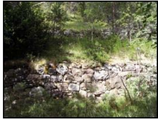
Figure 2.4. Actual state of masonry in the left bank
