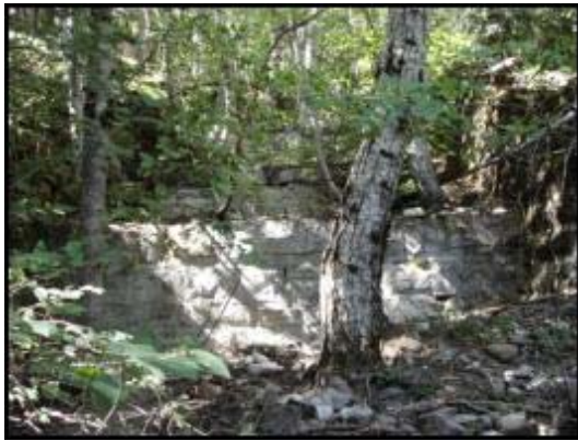
Figure 2.5. Channelization in the left bank
